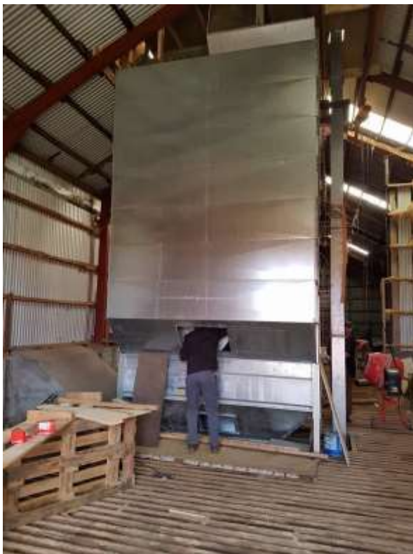
Figure 22. Installation of a dryer at Jaðar farm.
