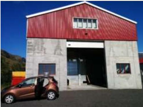
Figure 2. The new drying facility at Þorvaldseyri
