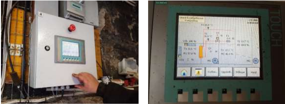
Figure 19. Monitoring unit for grain drying.
