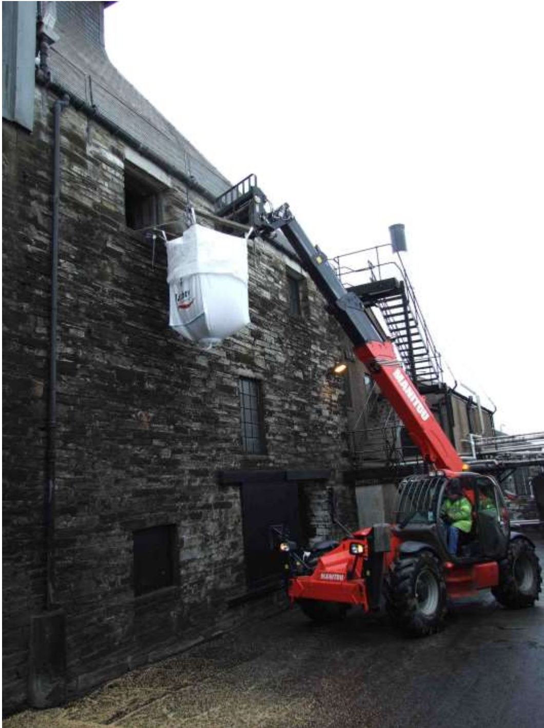
Photo 15. Unloading malt from the kiln.
